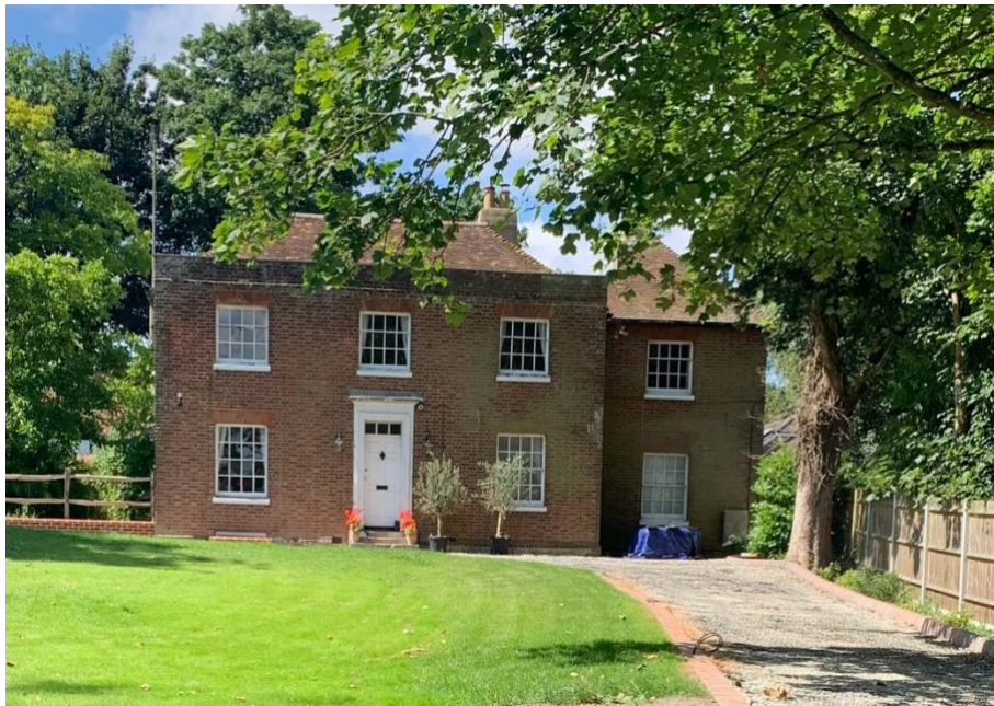
Parapet House ( photo taken in 2024)
